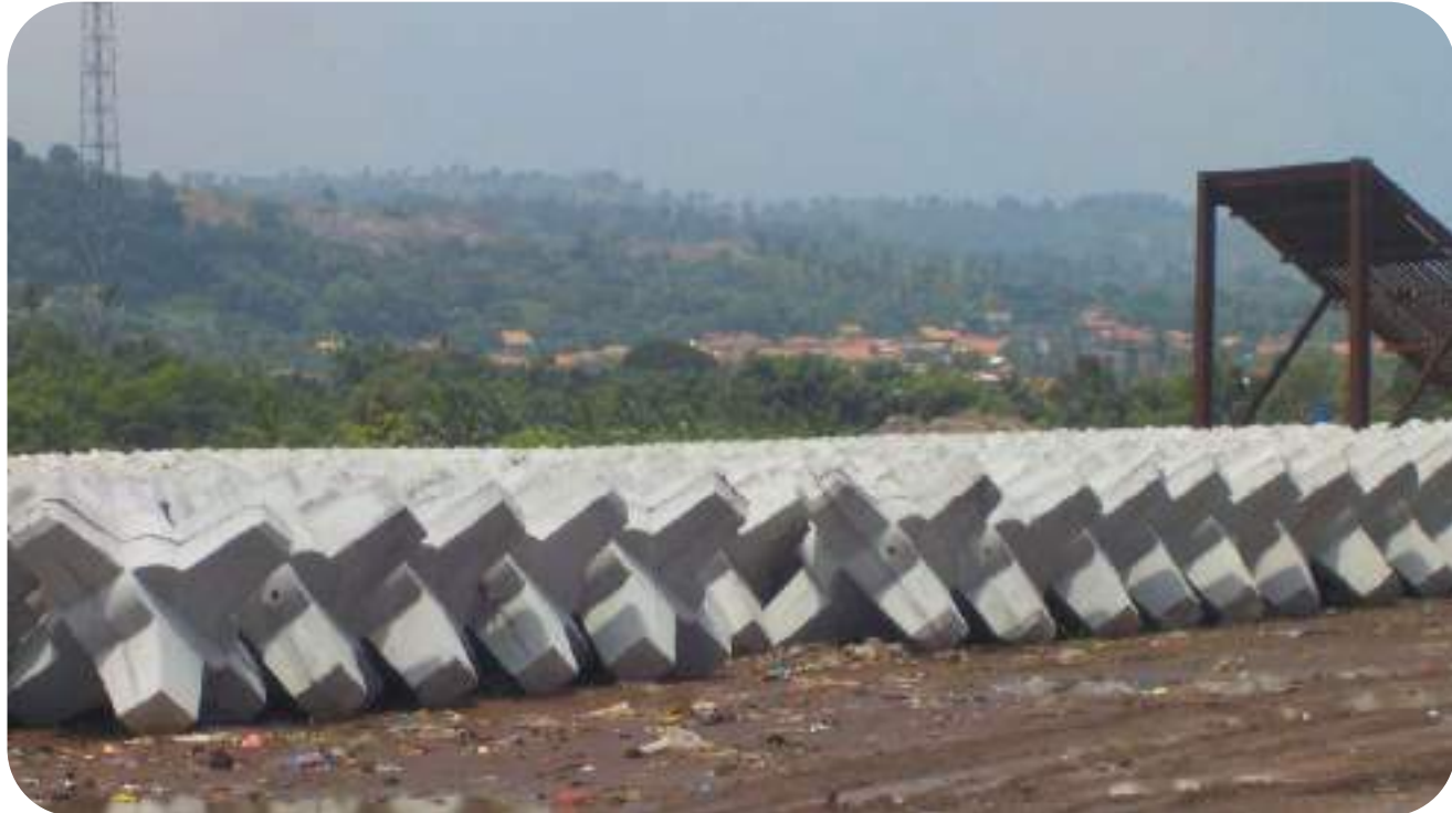
Breakwater Implementation “A-JACK” in Harbor.
