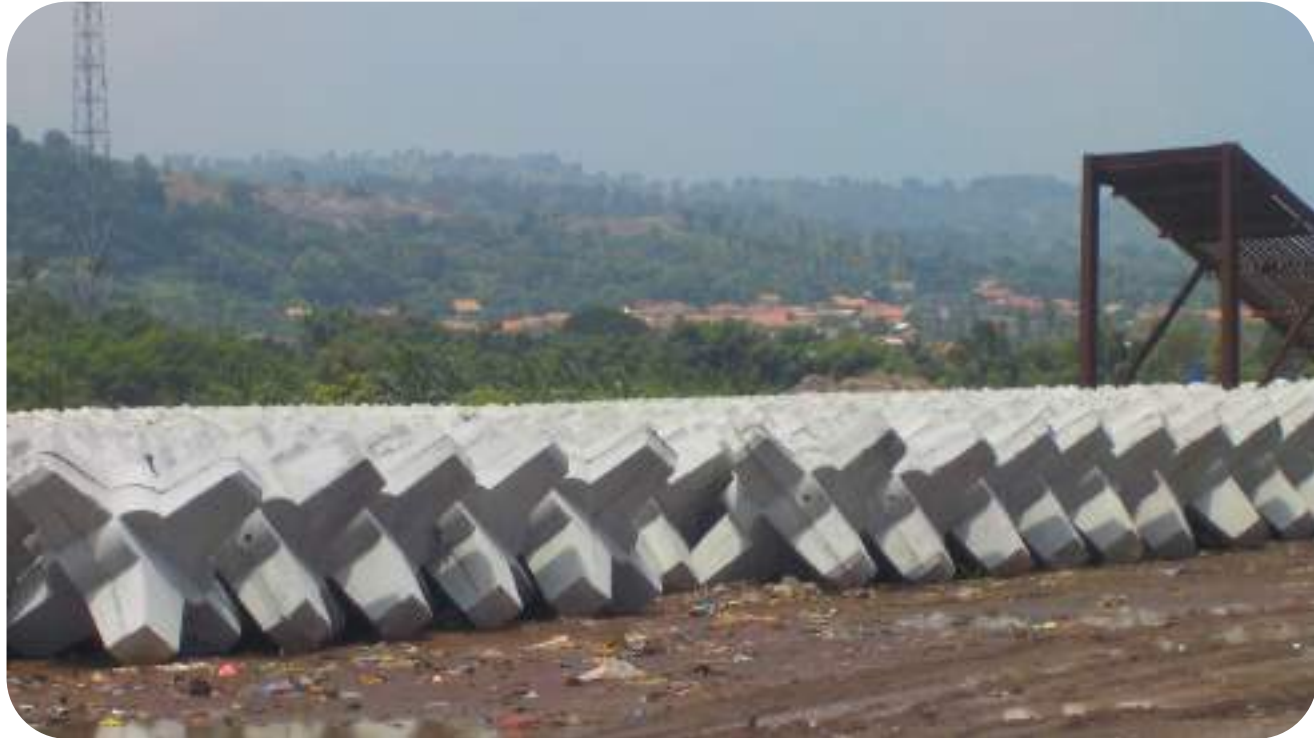
Breakwater Implementation “A-JACK” in Harbor.
