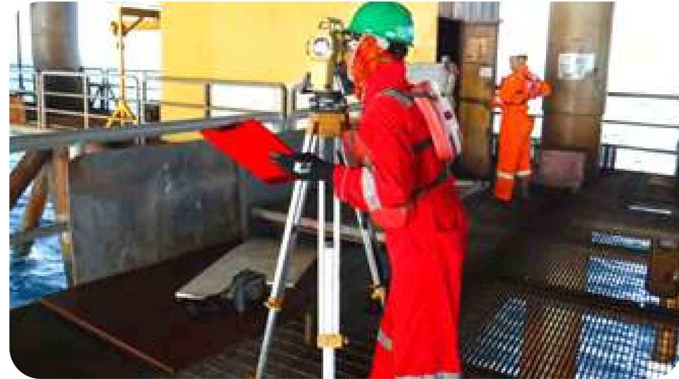
Engineering Services di Fasilitas Offshore
